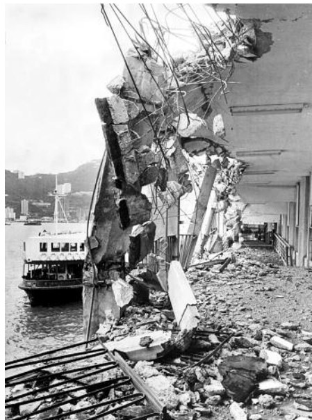
During Typhoon Hope one of Kowloon's two Star Ferry piers in Tsim Sha Tsui, was seriously damaged when the powerless 10,335grt Greek freighter Argonaut (ex Hazelbank) collided with the piers (above). Reportedly the ship lost its anchors and despite desperate efforts by the crew to avoid the Star Ferry piers, they were unsuccessful in their endeavour. The ship eventually came to rest hard up against Kowloon Public Pier, having sustained serious hull damage on her port side.
